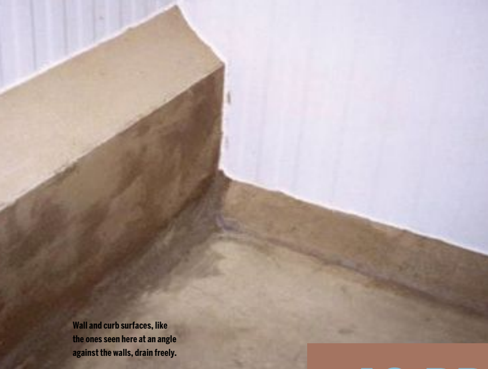
This plant has standing water on the floor, an uneven floor surface, and a 90 degree angle between the wall and the floor.
